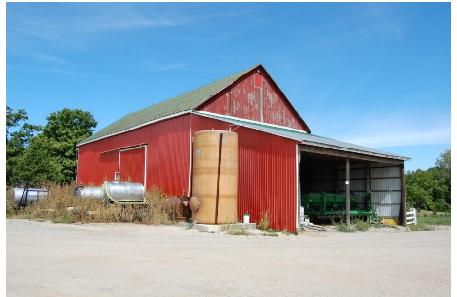
Figure 12 – Bank barn, viewed from south. (Photo: RHC, Aug 2012)
