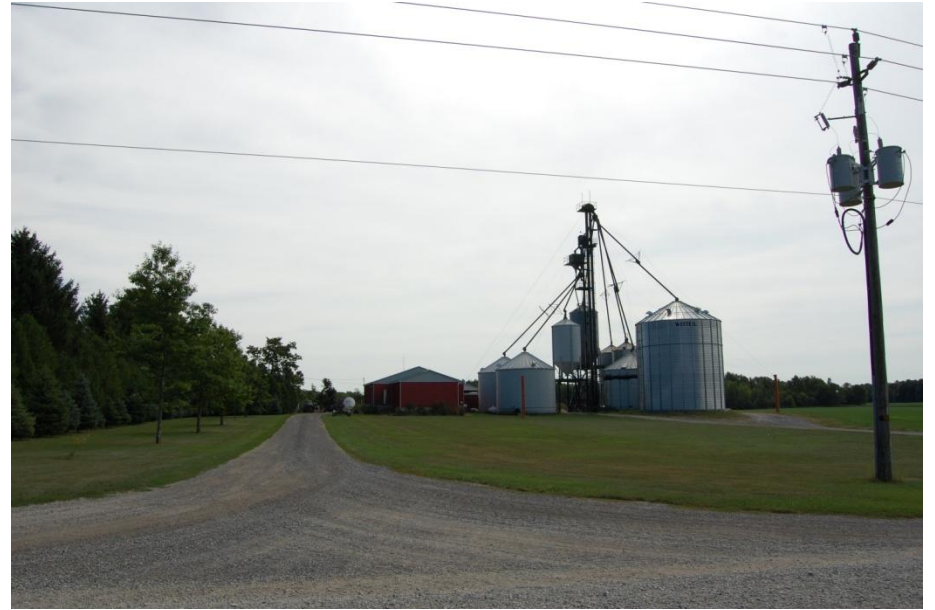
Figure 20 - View southeast from Union Drive. (Photo: RHC, Aug 2012)
