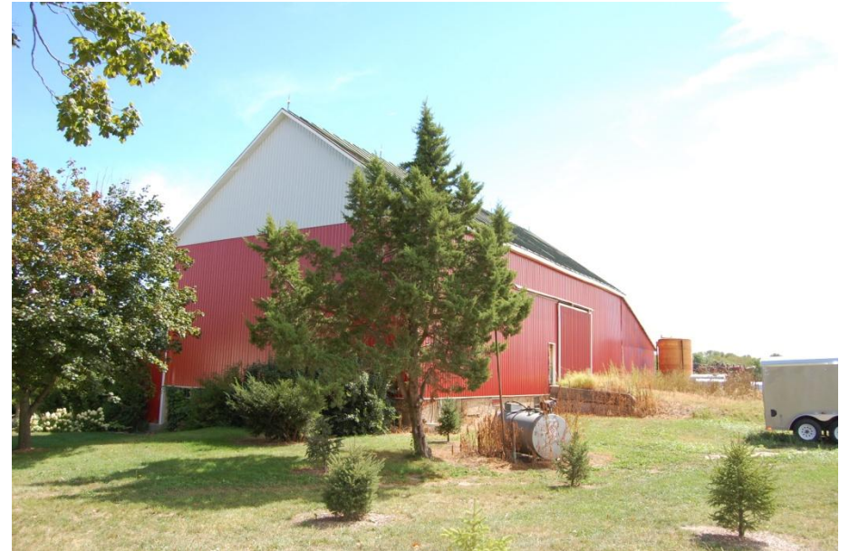
Figure 11 – Bank barn, viewed from west. (Photo: RHC, Aug 2012)
