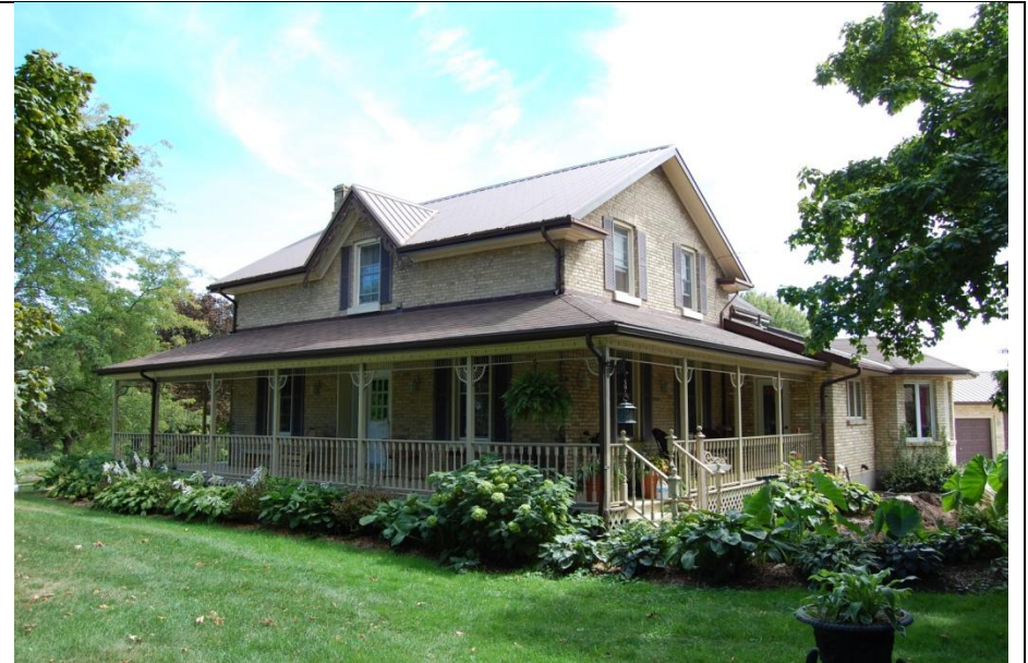
Figure 7 – Farmhouse, viewed from lane. (Photo: RHC, Aug 2012)
