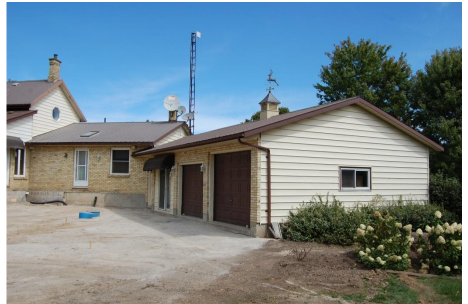
Figure 10 – Rear addition and attached garage. (Photo: RHC, Aug 2012)
