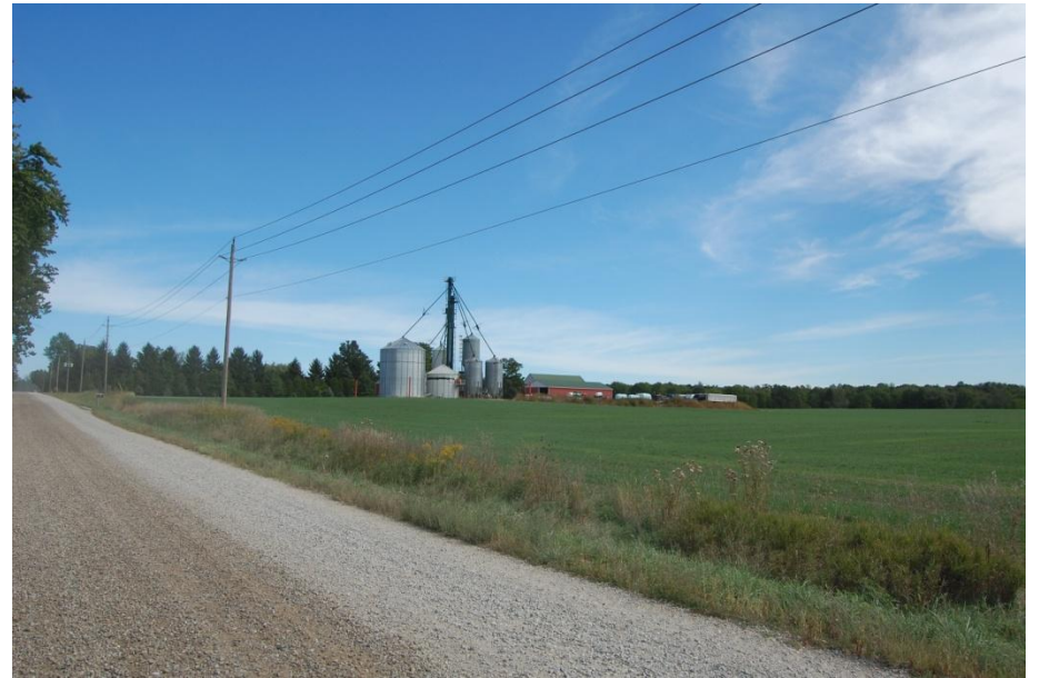
Figure 21 - View northeast from Union Drive. (Photo: RHC, Aug 2012)
